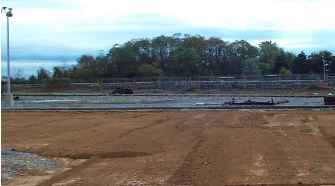
Figure 6. View of Treated Soil Awaiting Compaction and Surfacing
