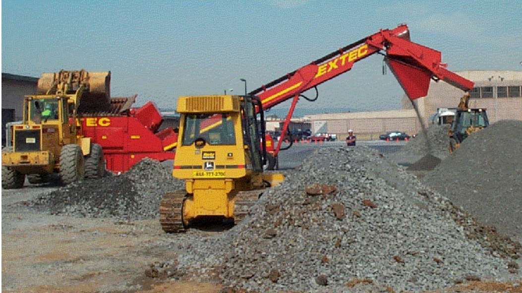
Figure 3. Soil Excavation and Screen Process
