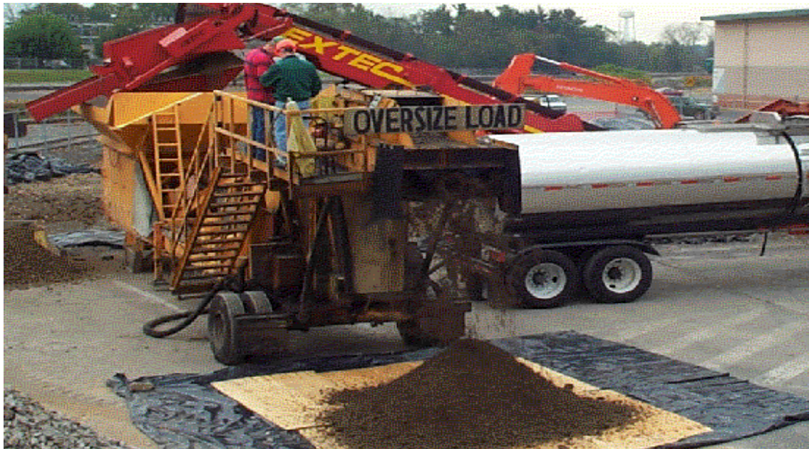
Figure 5. View of Pug Mill and Emulsion Tanker Truck
